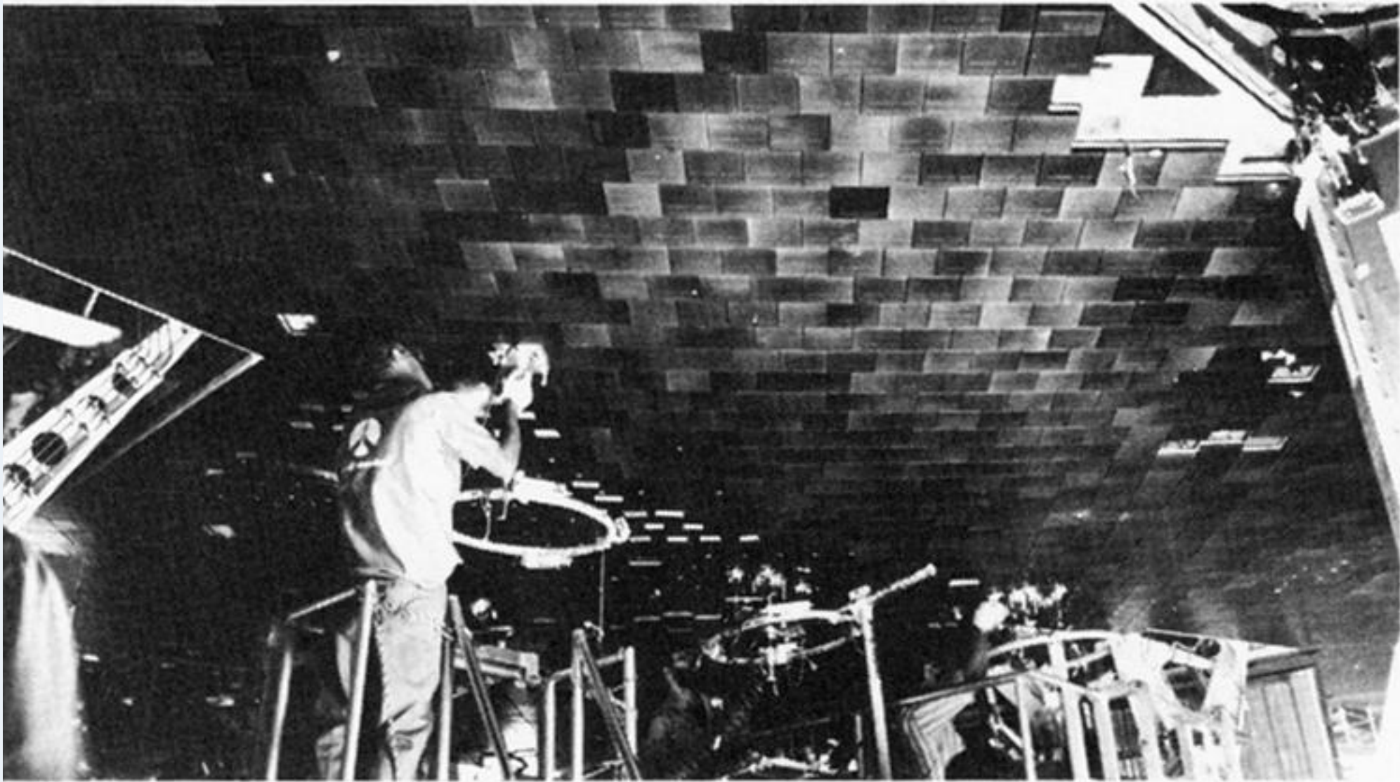
FIGURE 3. Tile installation.
